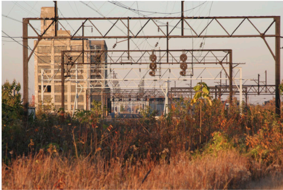
Reading Viaduct. Photo by Steve Weinik.
